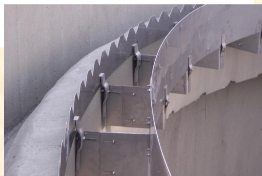
Stainless device Weir and floating dam / foam
